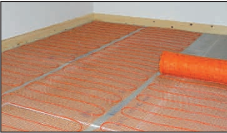
3mm twin-conductor heating cable sewn on to a self-adhesive mesh mat
